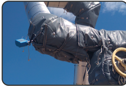
microTEMP attached with a band clamp out of insulation
