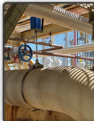
microPIMS I.S sensors installed using a band clamp
