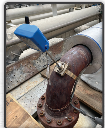
microPIMS I.S sensors installed using a band clamp
