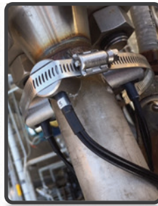
XD-101 and XD-301 attached with hose clamp
