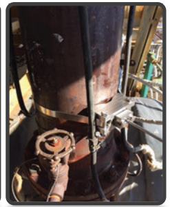
XD-201 probes attached with clamp
