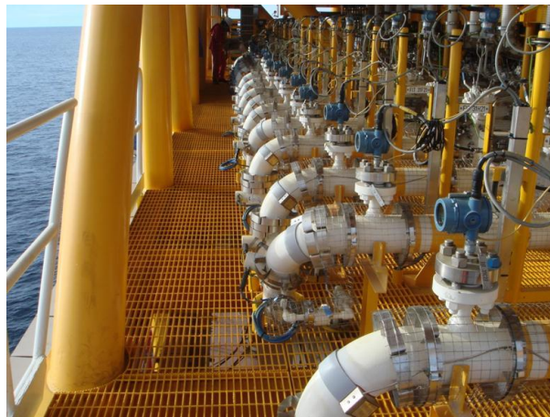
Figure 11: Installed transducer pads on critical elbows at an offshore production platform.
